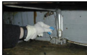
*Capillary tube (ferrous) identified*
